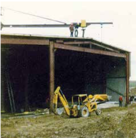
Allegheny Plant Construction - 1976
